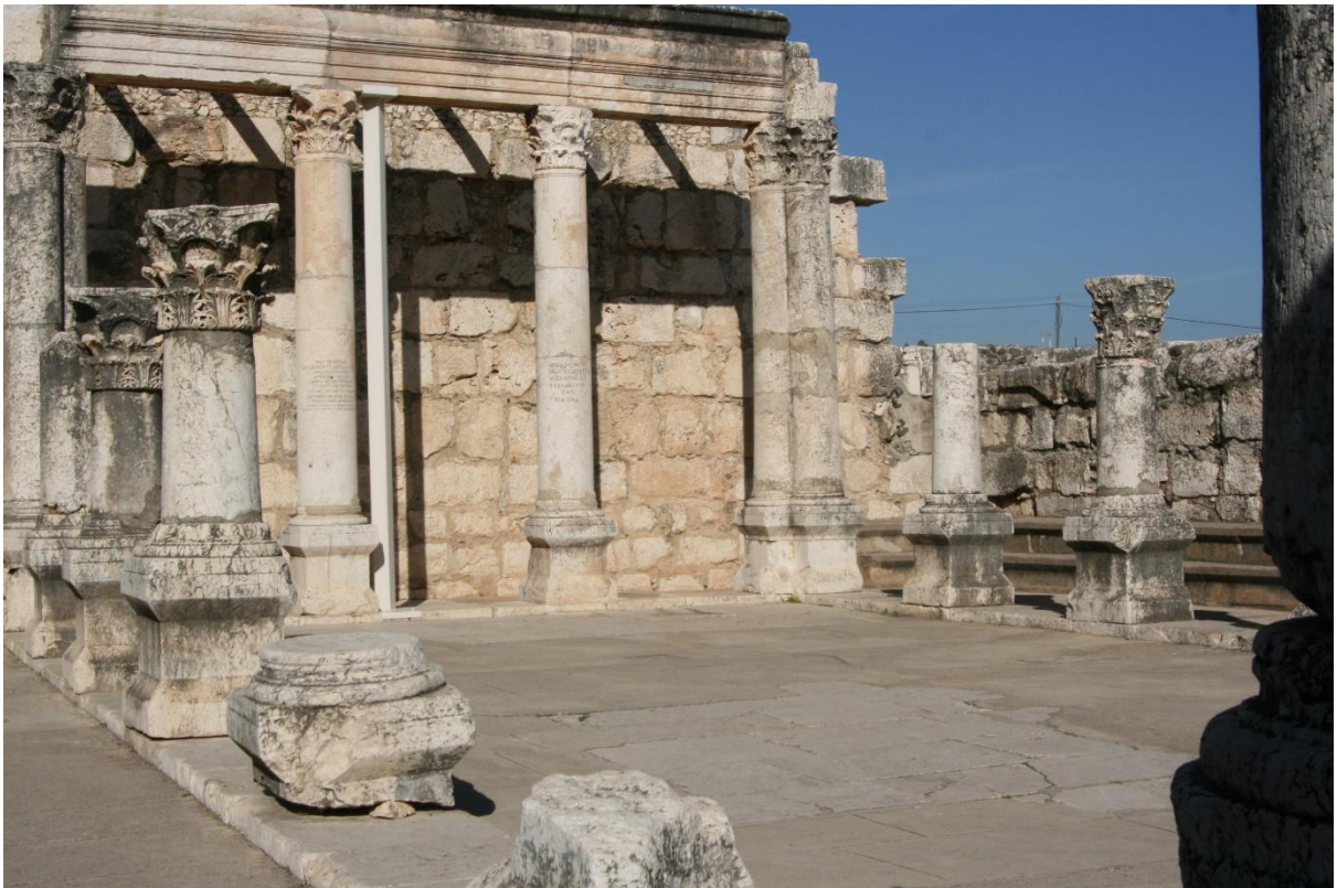
Section of the 4 th century CE Capernaum Synagogue built upon an earlier first century CE structure (synagogue?). Photo: © Michael Trainor, used with permission
